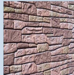
South Wall Replacement Following 2007 Collapse—Formlined, But Not Stained
